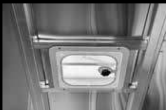
Roof vent in dressing room
